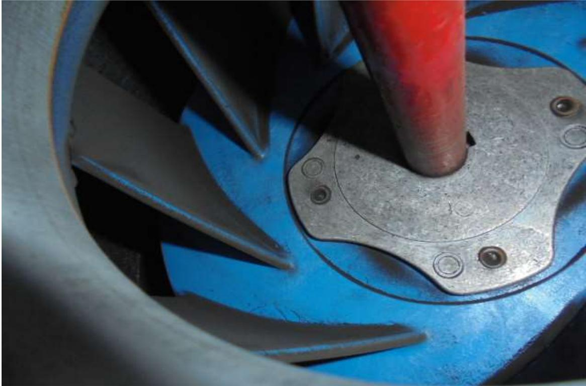
**Impacted Carbonaceous Dirt Deposit Observed on Fan Impellor Blades**
