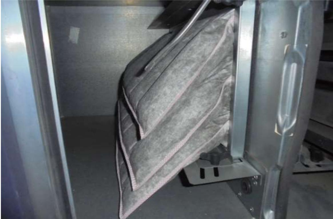
**Bag Filter Media Incorrectly Installed – Pockets Should Have a Vertical Orientation**
