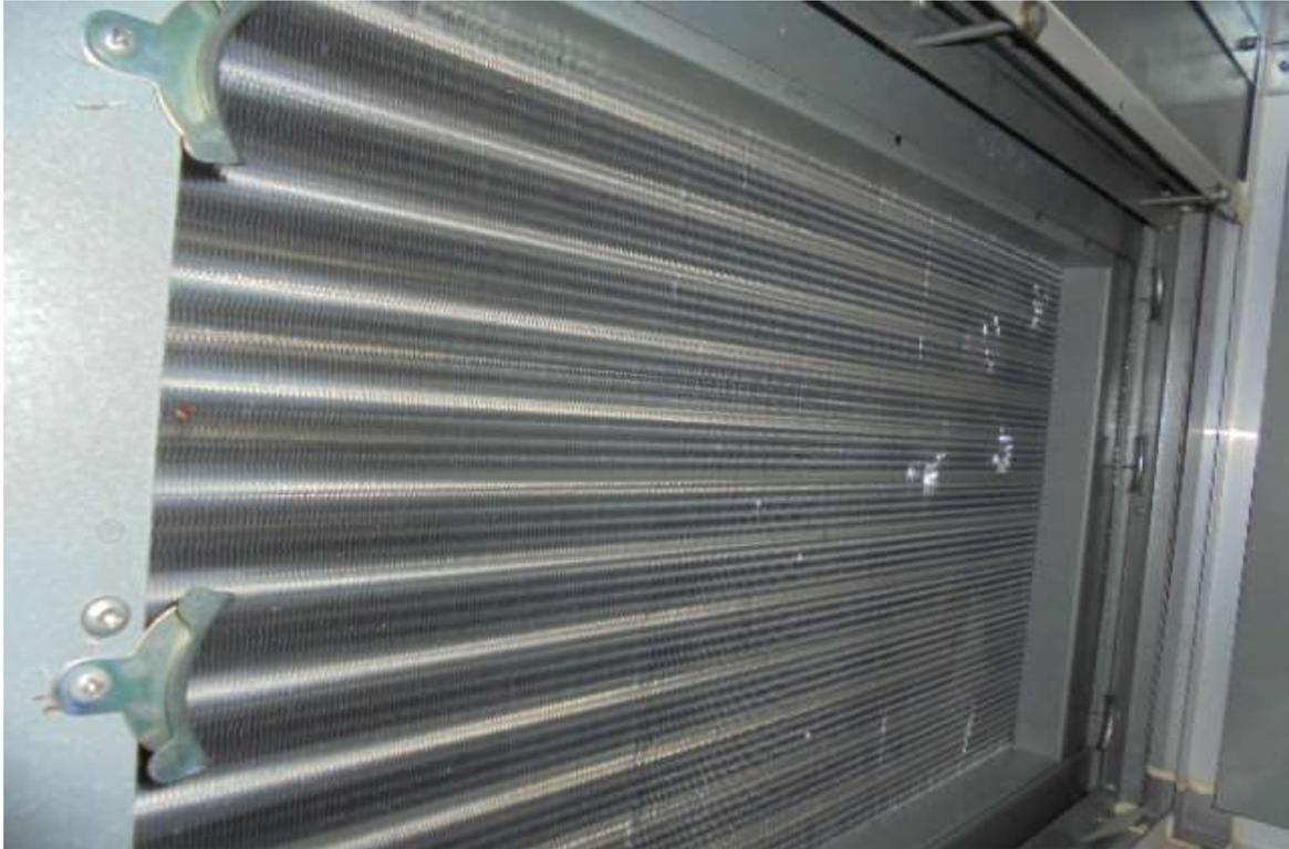
**Minimal Mechanical Damage Only Noted on Upstream Face of Battery Heat Transfer Fins**
