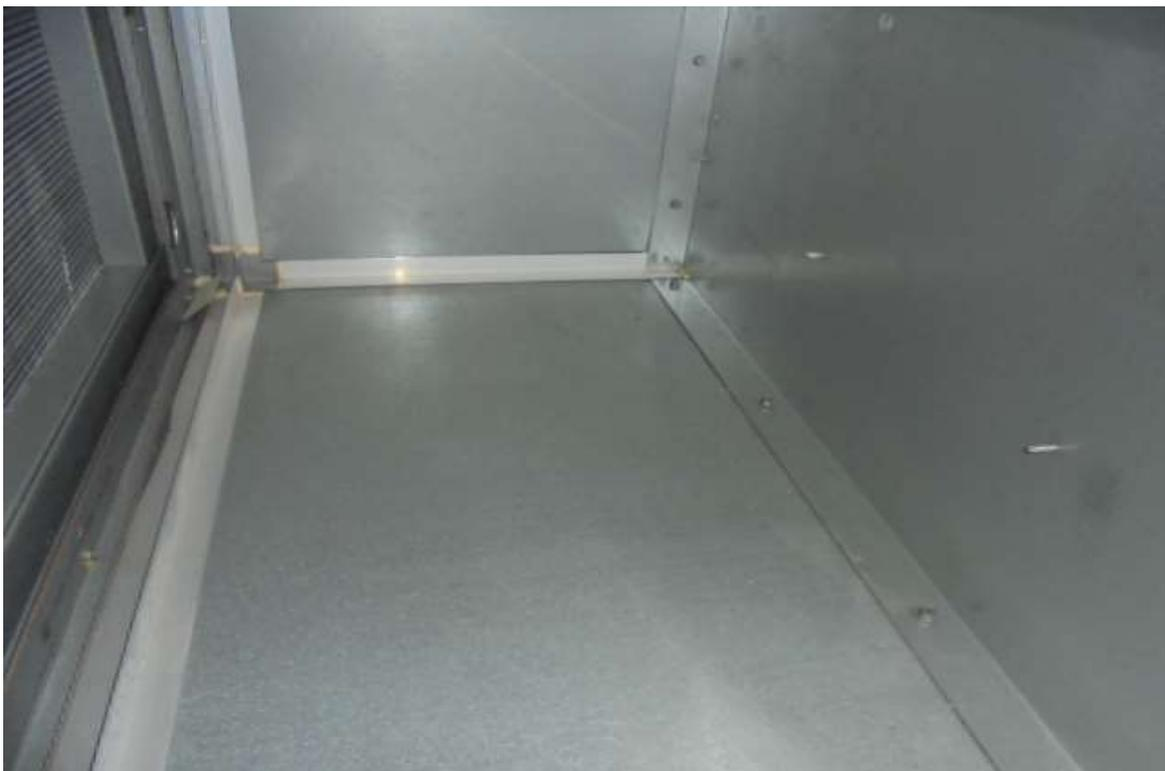
**Good Hygienic Condition With Minimal Particulate Deposit Noted Within Conditioning Section**
