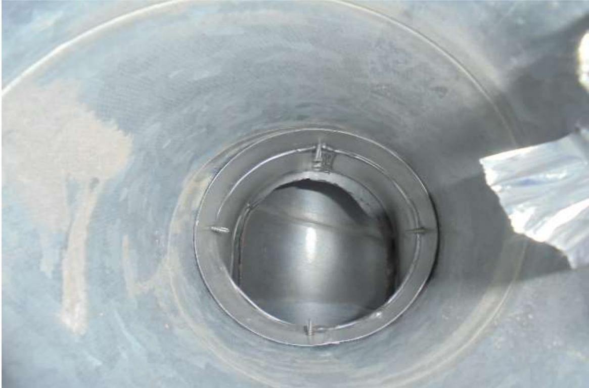
**Minimal Particulate Deposit Noted on Internal Surfaces of Distribution Ducting**
