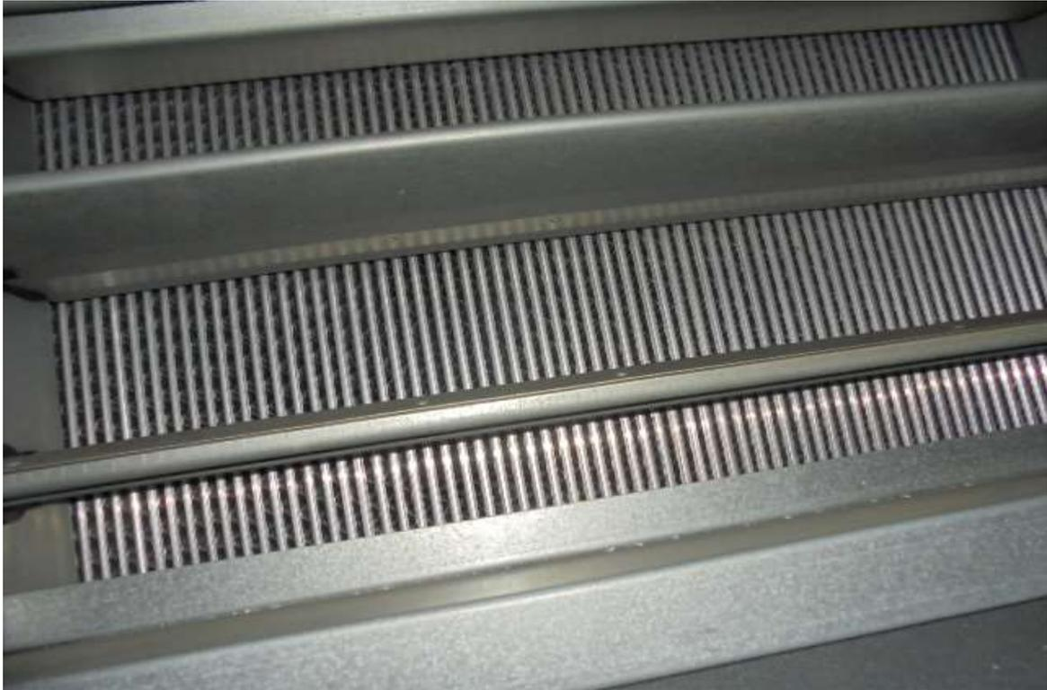
**Good Mechanical and Hygienic Condition of Upstream Face of Recuperator Components**
