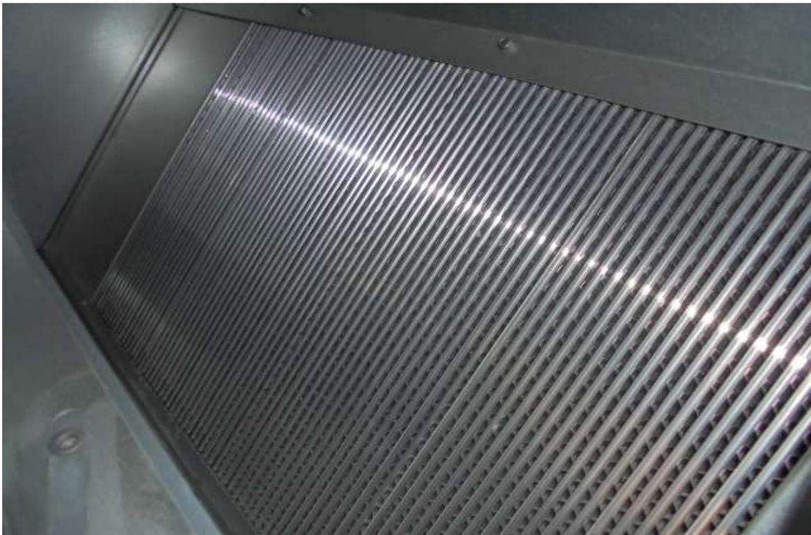
**Exhaust Air Side of Recuperator Also Found to be in Good Hygienic and Physical Condition**
