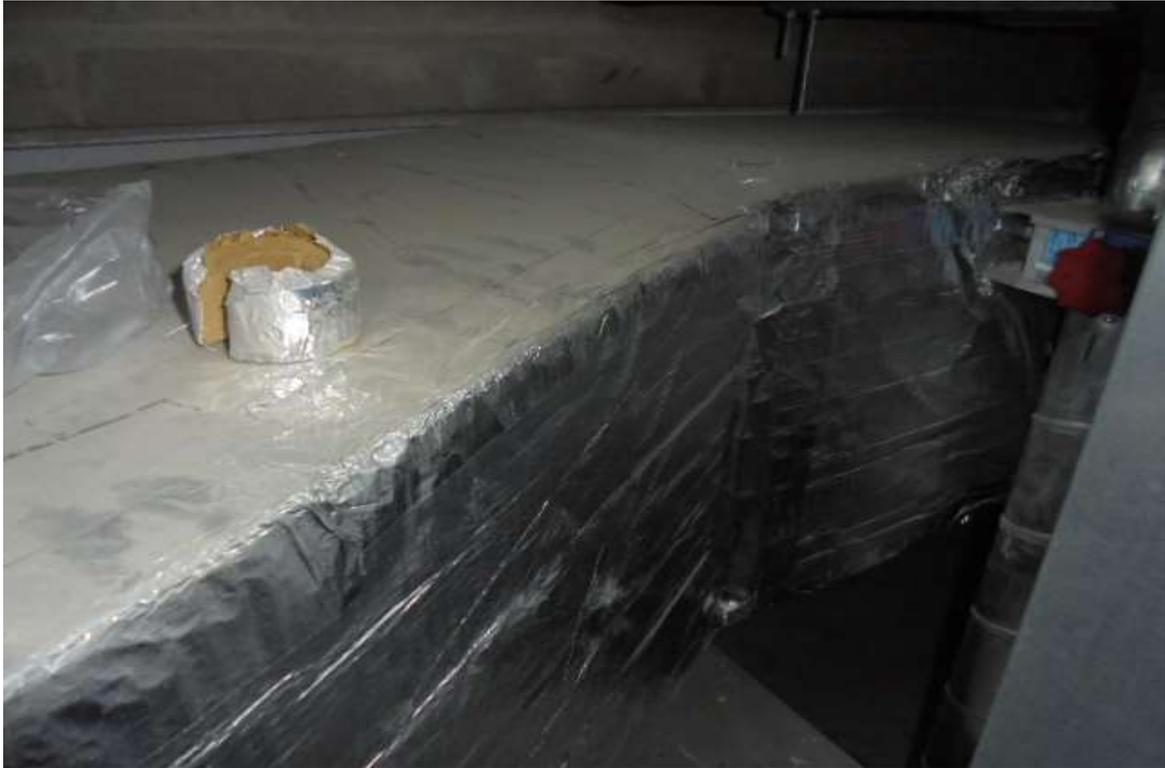
**No Access to F/A Ducting Severely Restricting Opportunity for Inspection and Test, or The Implementation of Hygienic Maintenance**
