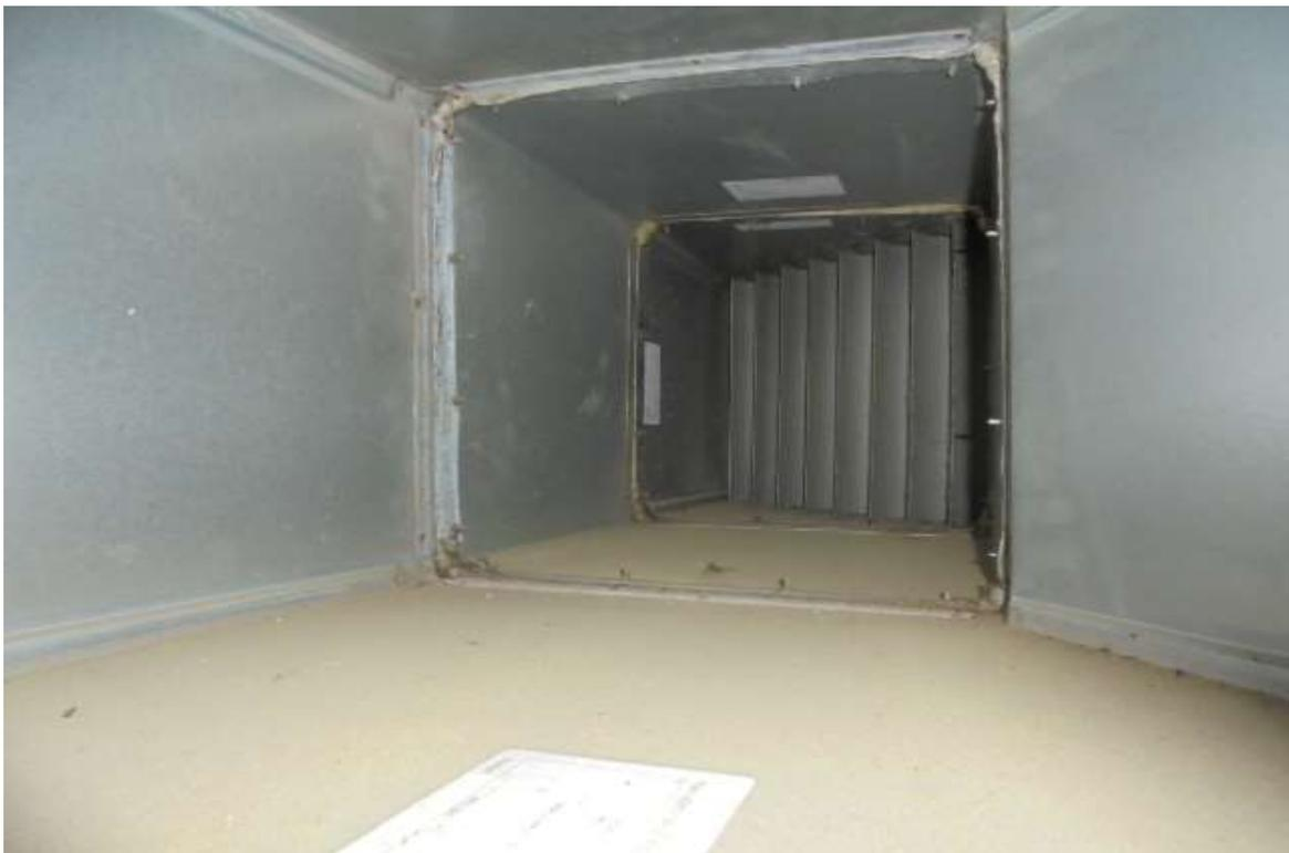
**Moderate to Heavy Particulate Deposit on Horizontal Surfaces of Fresh Air Intake Ducting**
