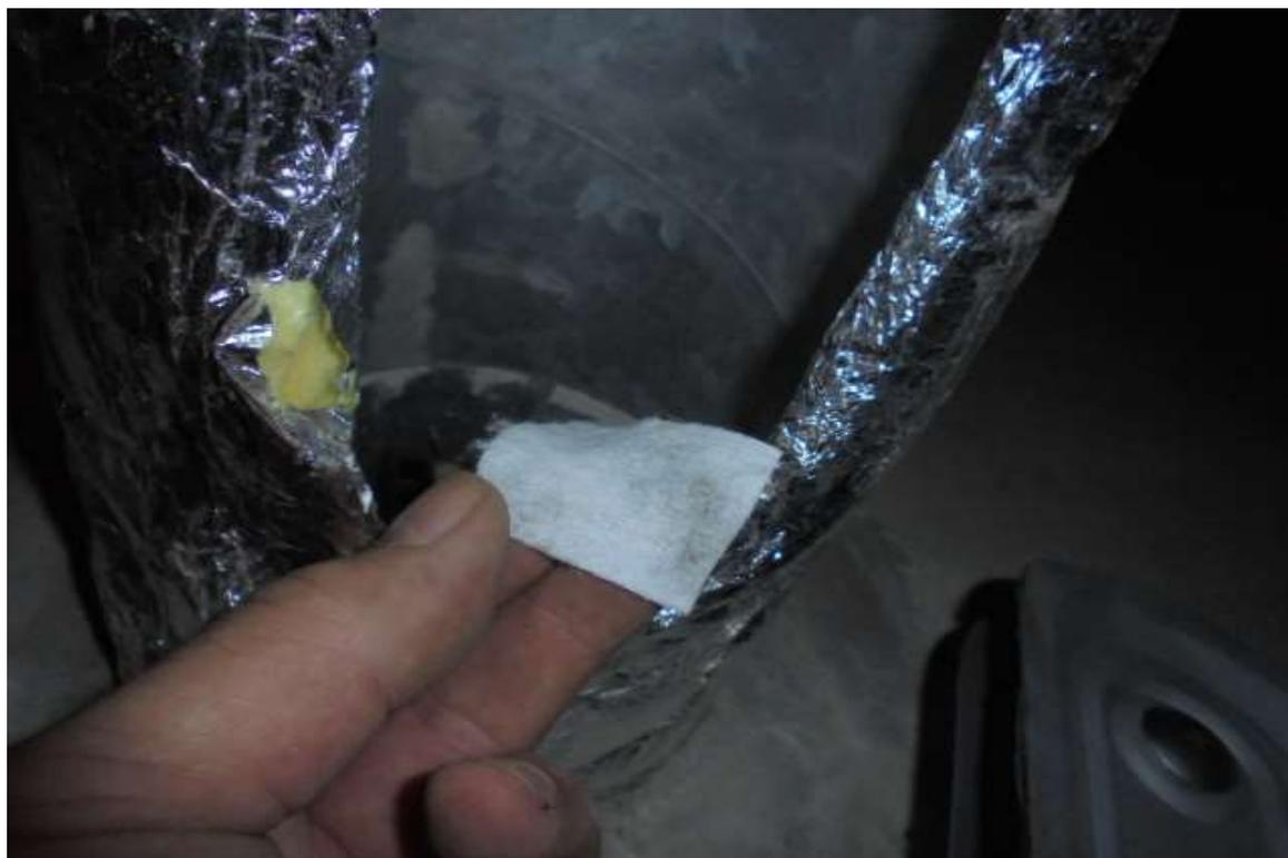
**Sample Retrieval from Distribution Ducting Confirming Particulate Deposit to be Light**
