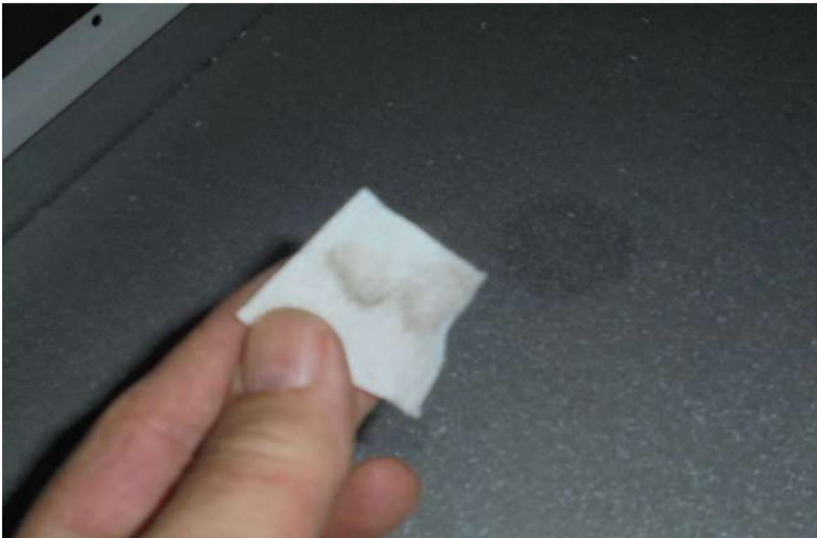
**Light Particulate Deposit Noted on Floor of Conditioning Sections**
