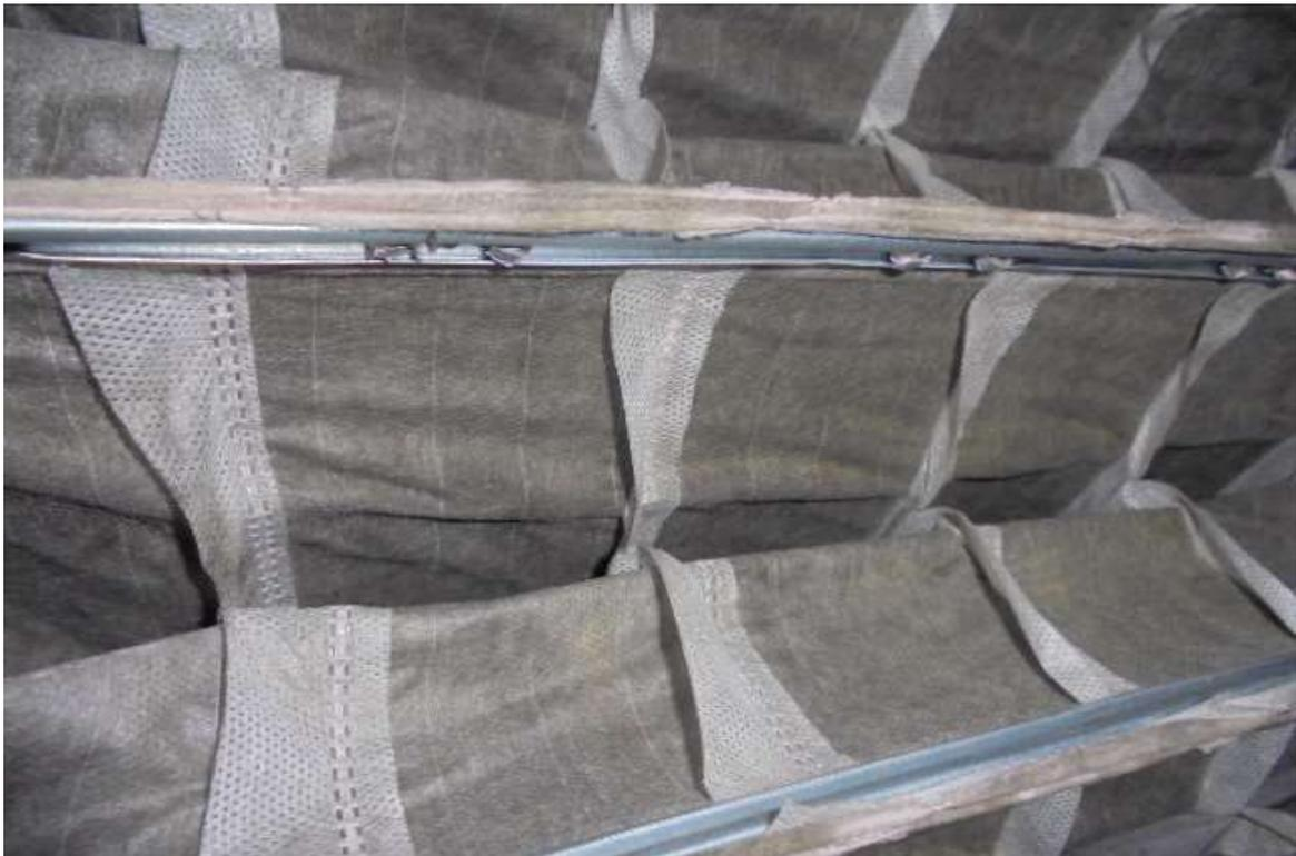
**Moderate to Heavy Particulate Load on Secondary Filter Media Noted**
